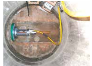
BURSTFIX 200 inside the manhole
